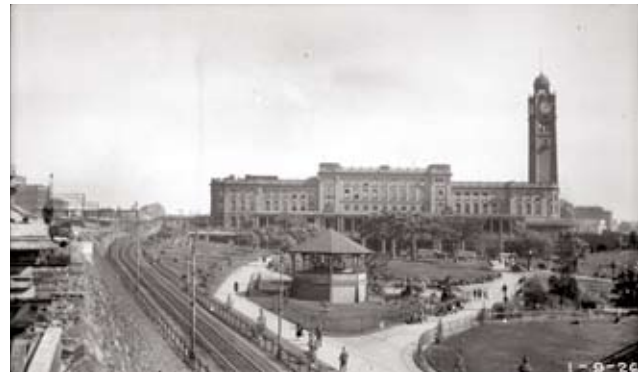
Central Station and Belmore Park, R C Robertson, 1926, printed from glass plate negative, State Records NSW
